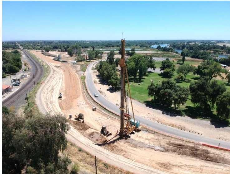
Marysville Ring Levee Project, CA
